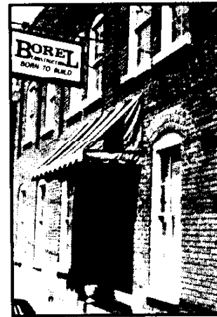
Borel's historic exterior
