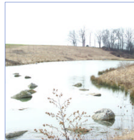
Regional stormwater detention facility located on the campus of Virginia Tech.
